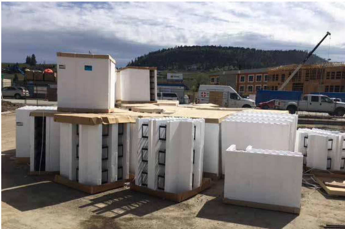
Insulated Concrete Forms were used in the foundation and walls
